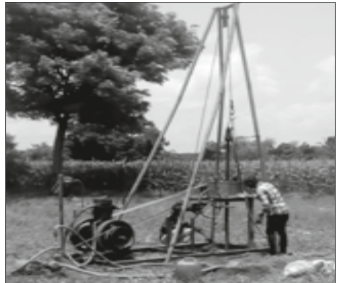
Fig. 3 Drilling using Calyx Drill Rig
