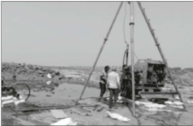
Fig. 5 Drilling Using Hydraulic Rotary Drill Rig
