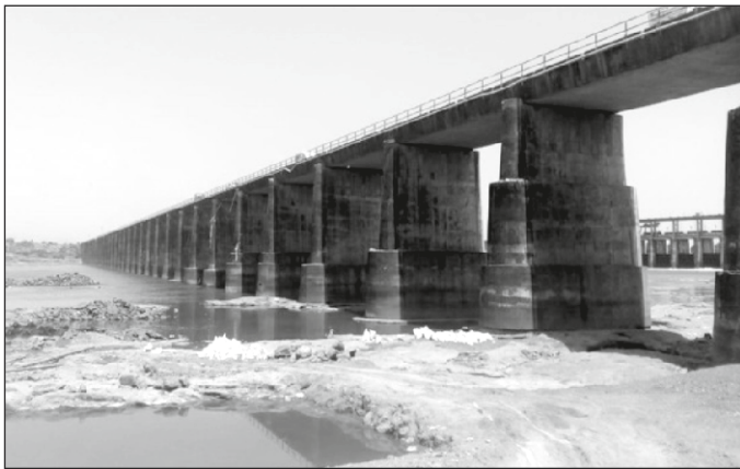
Fig. 2 Rock Exposed Along Alignment Adjacent to Existing Bridge.
